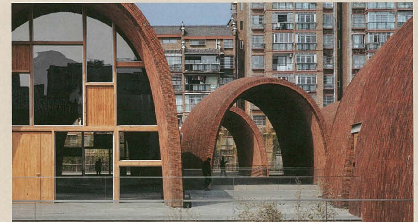
The brick vaults at Studio Zhu-Pei's Imperial Kiln Museum, Jingdezhen, China, are based on the form of a traditional kiln.
