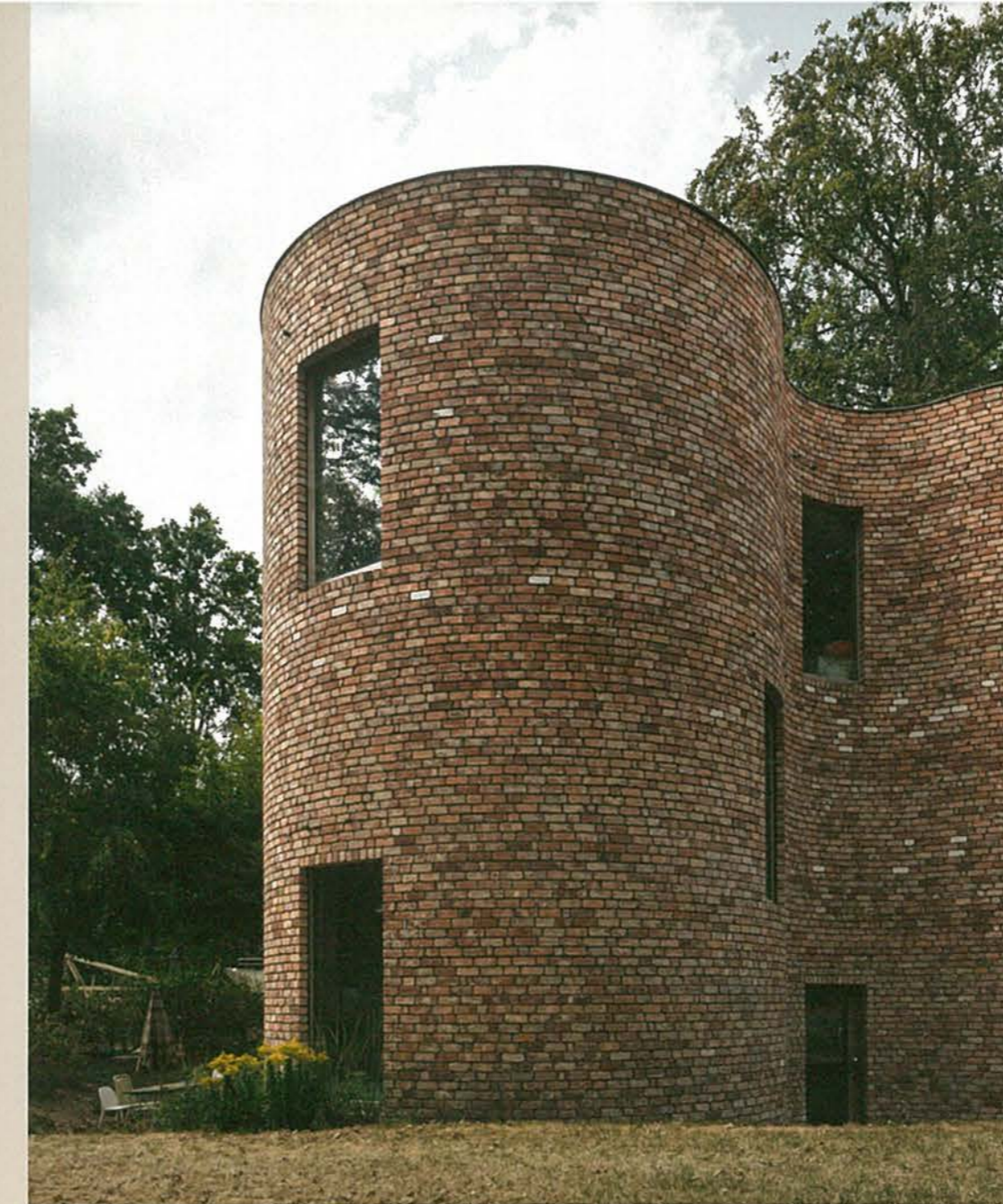
The curvaceous brick forms of Studio Zhu-Pei's Imperial Kiln Museum, Jingdezhen, China (opposite), and BLAF Architecten's gJG House (above).
