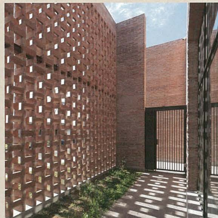
At Casa Joven in San Francisco, Argentina, the architects have used a perforated brick screen to distance the house from the street.
